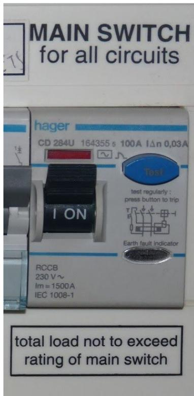
If a fault occurs, or a person gets an electric shock, a small amount of current flows from Live to Earth – this is the residual current. The current in the Neutral wire is less than the current in the Live wire. A Residual Current Circuit Breaker (RCCB) detects the small difference in current in the Live and Neutral and disconnects the electrical supply. An RCCB is very fast, disconnecting the supply in just a few milliseconds.
